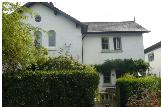
New Windows in Original Openings
